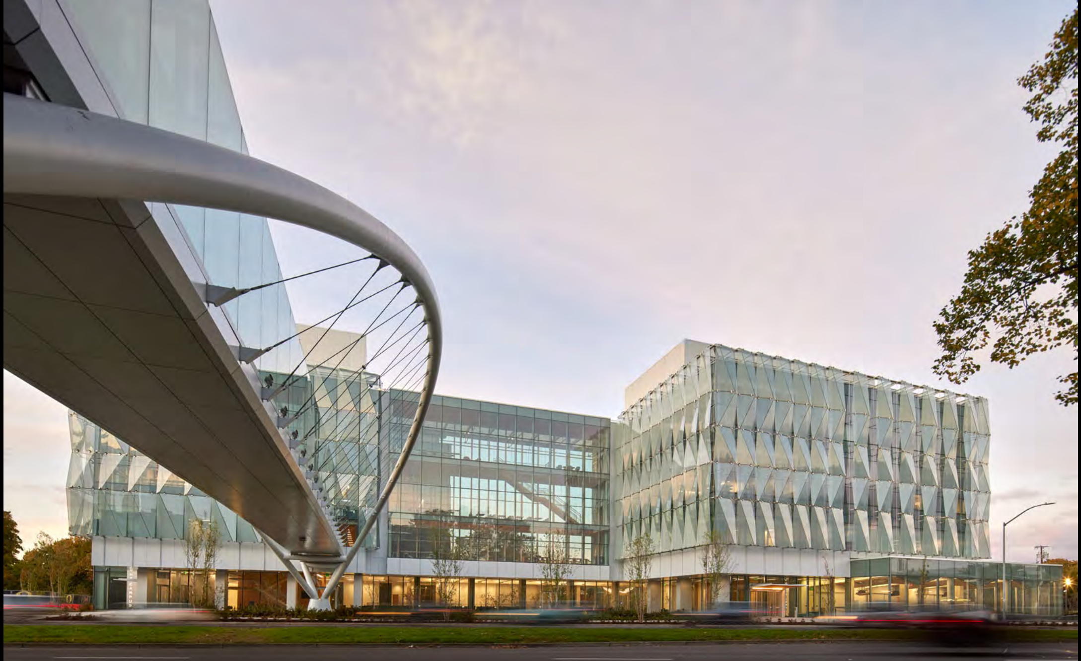
View skybridge, connector, and east tower from Franklin Boulevard
